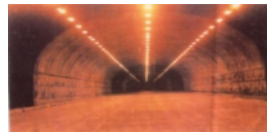
Fig.1. Present Lightening in the Tunnel using Sodium Vapour Lamp
