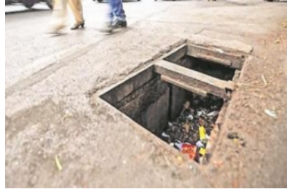
Fig 2: Dinesh Jatholiya falling into Manhole
